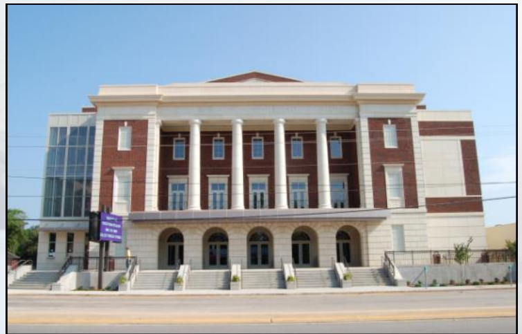
Township Auditorium After Renovations
