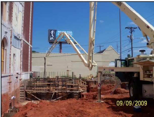
Exterior View of the Construction of Township Auditorium
