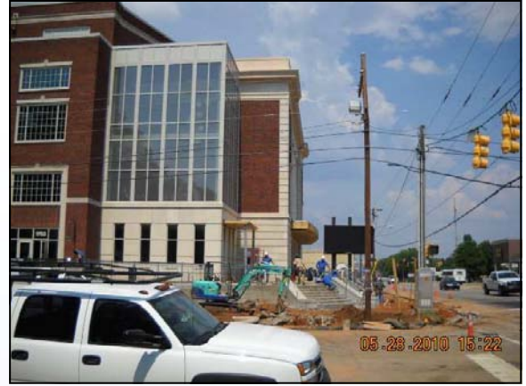
Exterior Facade of the Completed Township Auditorium
