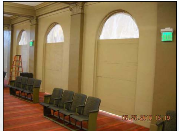
Newly Renovated Interior Features of the Township Auditorium
