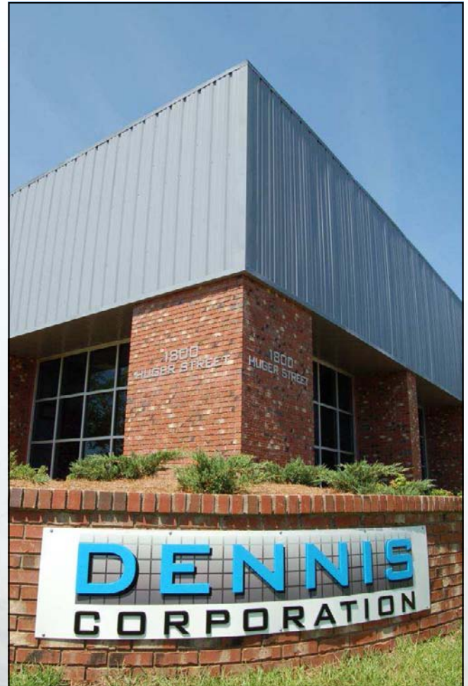
New Dennis Corporation Headquarters
