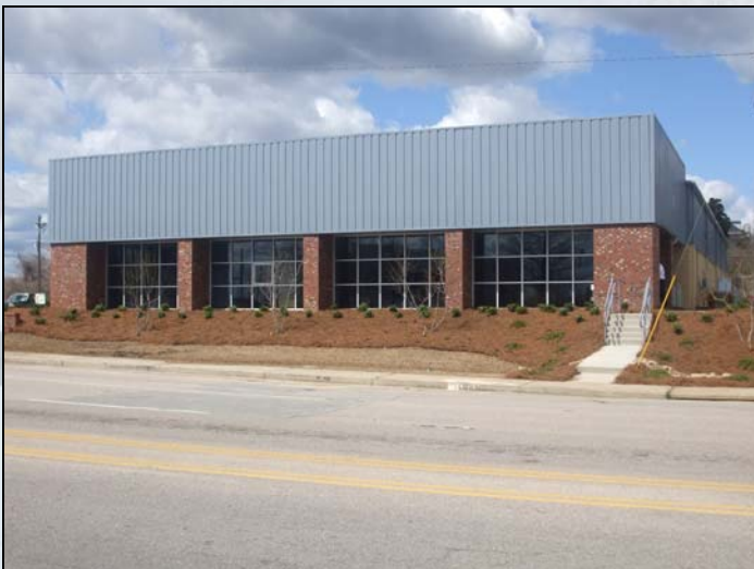
The Front of the Completed Building
