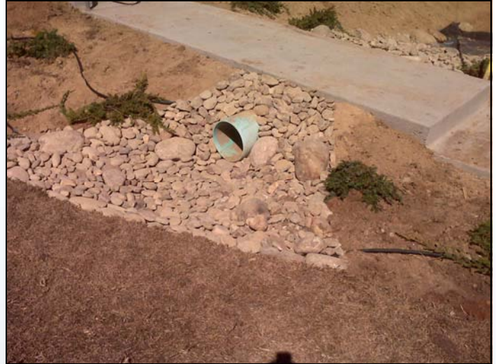
Stones Placed in Drainage Area are Both Decorative and Functional
