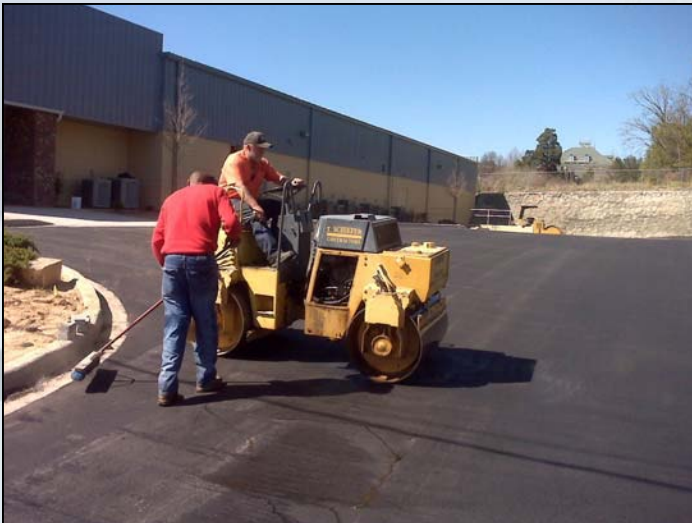
Newly Paved Parking Lot
