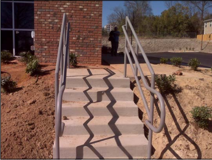
Rails Installed on Front Stairs
