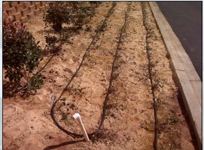
Irrigation Drip Lines Laid for Landscaping
