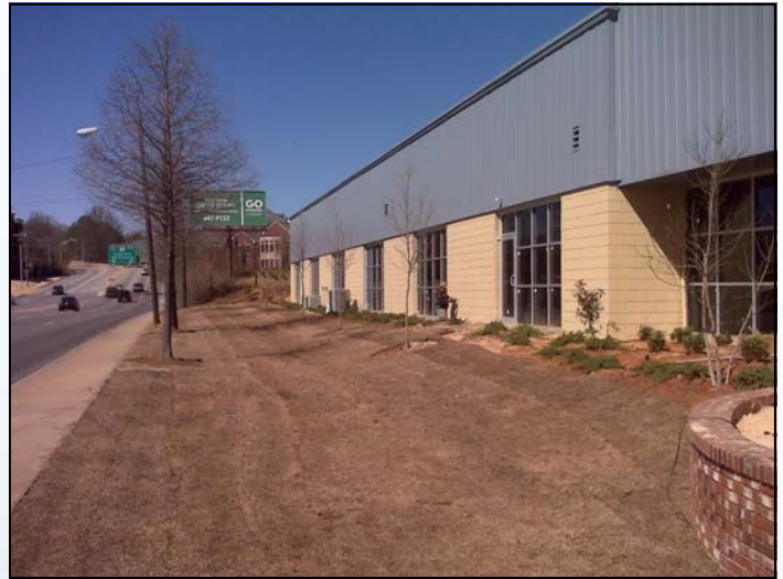
Painting and Exterior Work Nearing Completion
