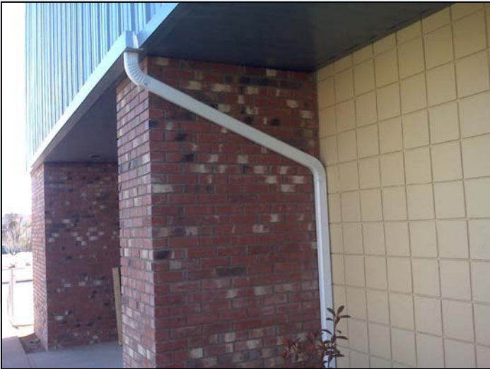
Gutter Installed Over Front Door
