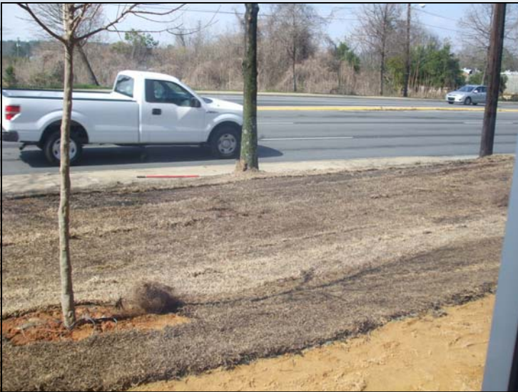
Grass is Put Down Outside of the New Building March 3, 2010
