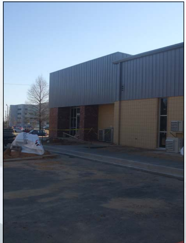
New Exterior Painting of the Metal Roof February 26, 2010
