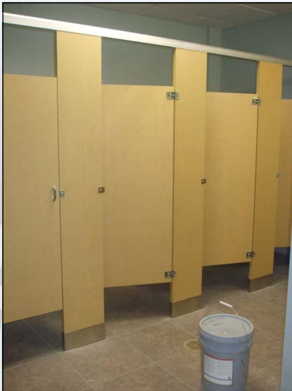
Installation of Bathroom Stalls Complete February 26, 2010
