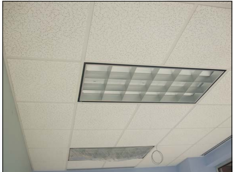
Lighting Fixtures Were Installed February 26, 2010
