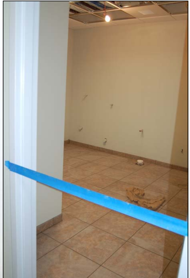
Tiles Installed in Men's Bathroom February 17, 2010
