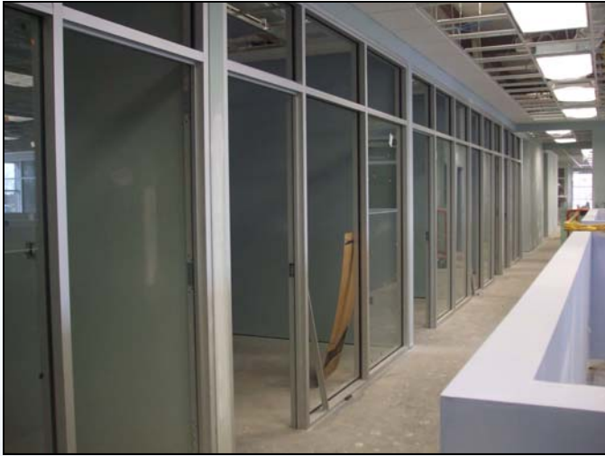
An Inside View of the Offices and Hallway February 19, 2010
