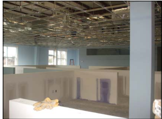
Cubicles and Offices in the Back of the Building February 8, 2010
