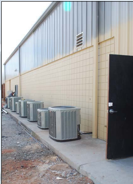
Painting Began on the Outside of the Building February 11, 2010
