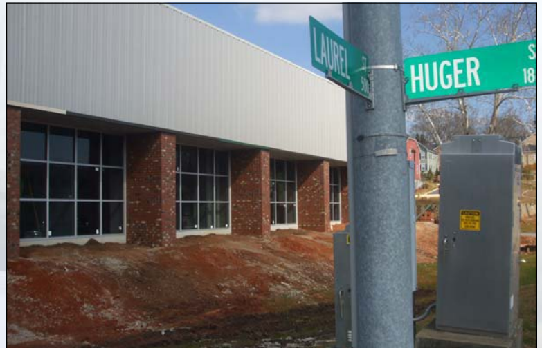
The Outside of the Building Facing Laurel Street February 8, 2010
