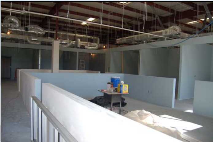
Construction on the Back Offices February 1, 2010
