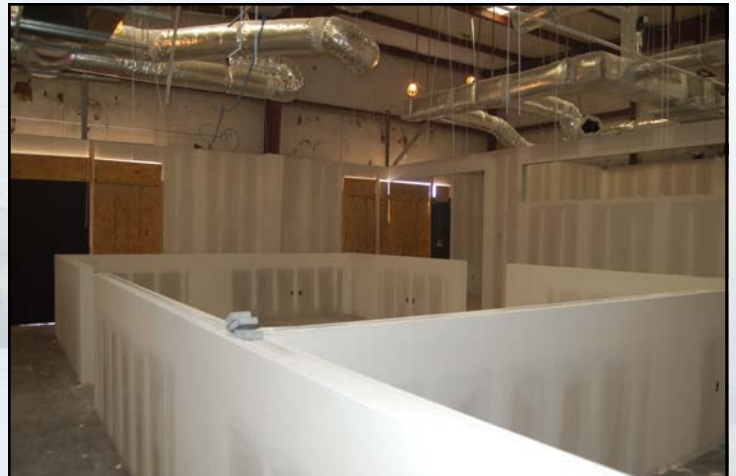
Cubicles and Offices in the Back of the Building January 26, 2010
