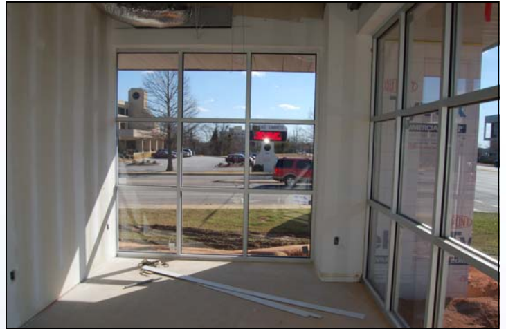
A View of Laurel Street from Inside January 26, 2010
