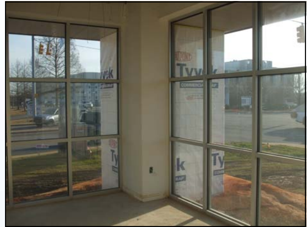
Newly Installed Windows January 22, 2010
