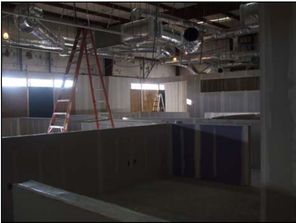
Offices in the Back of the Building are Constructed January 20, 2010
