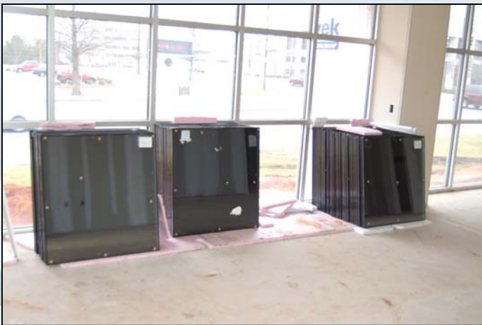
New Window Panes January 22, 2010
