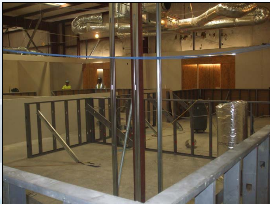
Cubicle Construction January 15, 2010
