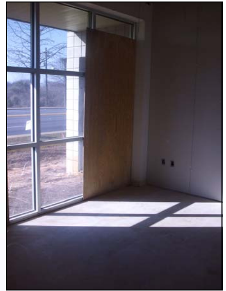
Window Installation January 15, 2010
