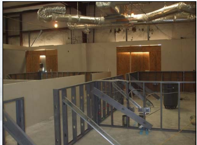
Cubicle Walls Begin to be Constructed January 15, 2010
