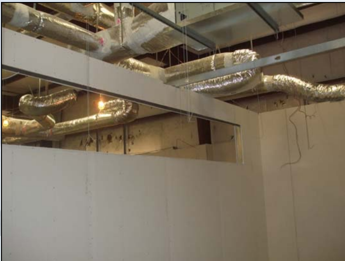
Air-Conditioning Units Continue to be Installed January 14, 2010
