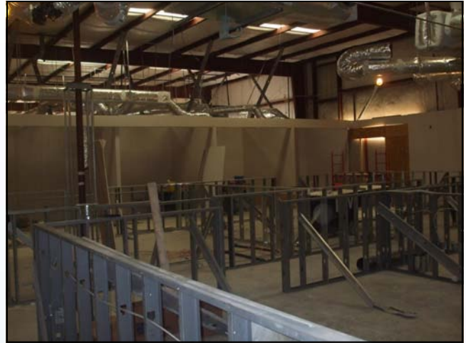
Cubicle Walls Begin to be Constructed January 14, 2010
