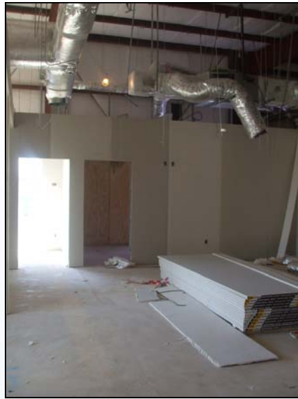
Installation of Drywall Continues January 15, 2010
