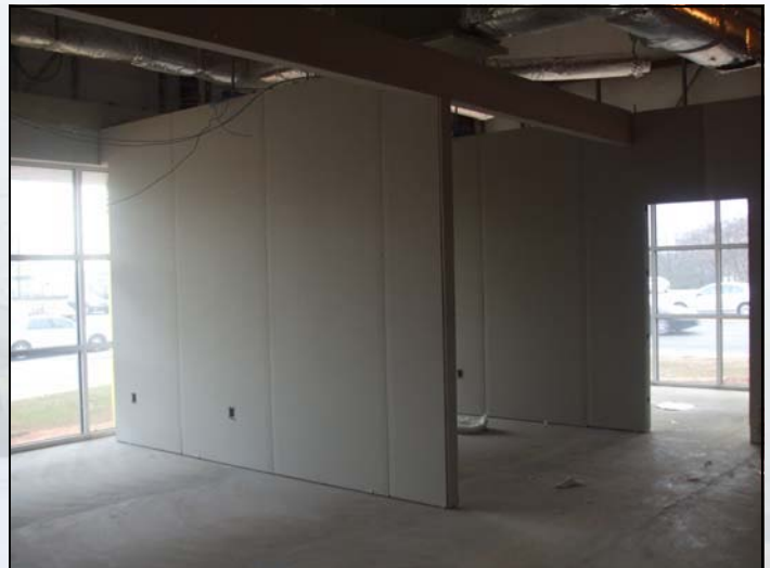
Electric is Installed January 7, 2010
