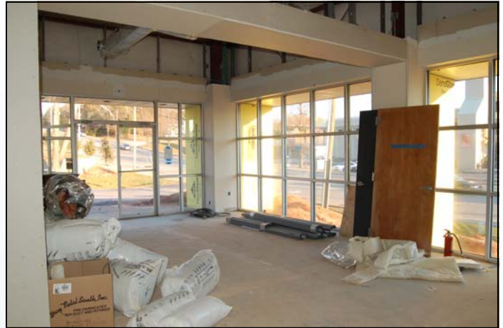
Renovations Continue on the Inside January 4, 2010
