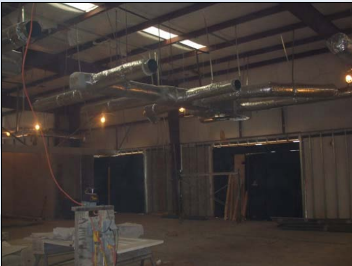
Air-Conditioning Units Continue to be Installed January 7, 2010
