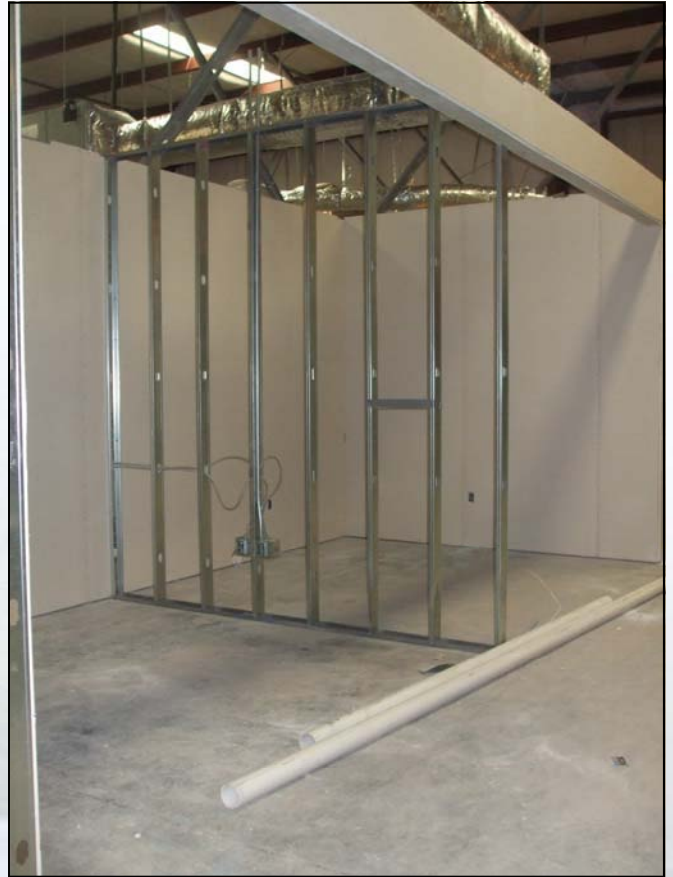
Inside Construction December 31, 2009
