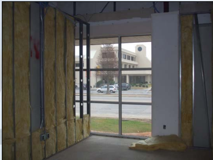
Insulation Installed December 31, 2009
