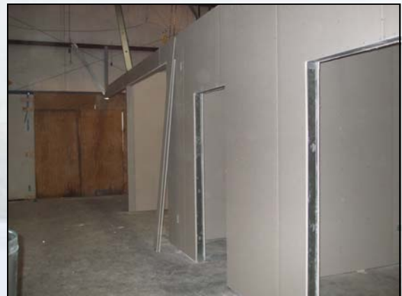
Walls are Completed December 31, 2009
