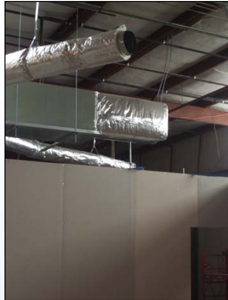
Air-conditioning Units Begin to Be Installed December 31, 2009
