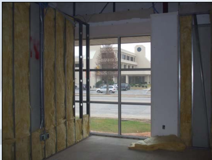
Insulation Installed December 31, 2009
