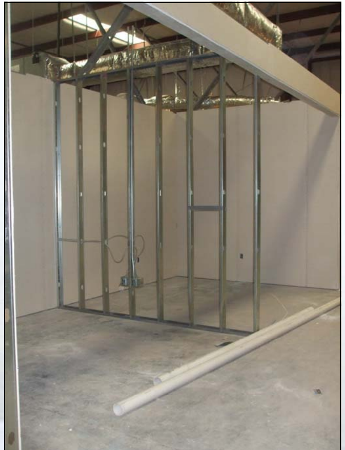
Inside Construction December 31, 2009
