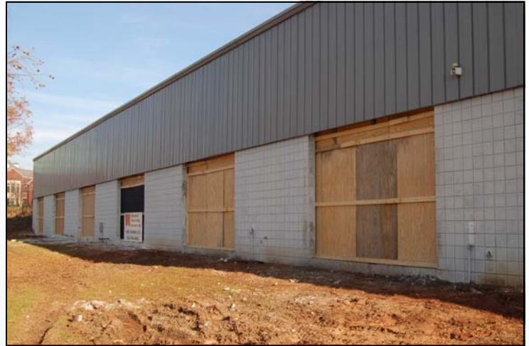
Preparing to Install Windows December 23, 2009
