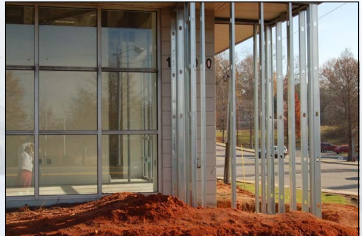
Preparing the Outside of the Building December 23, 2009
