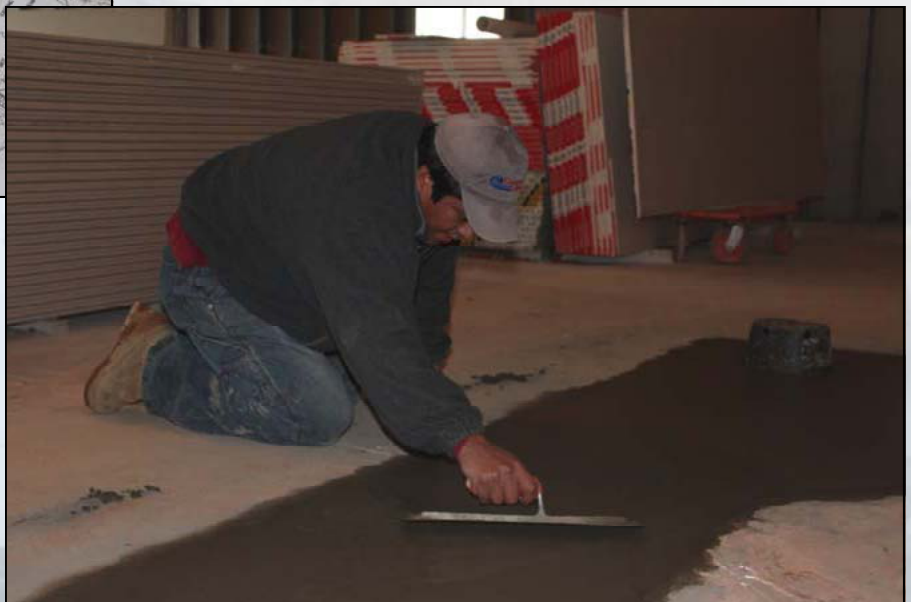
Leveling Concrete
