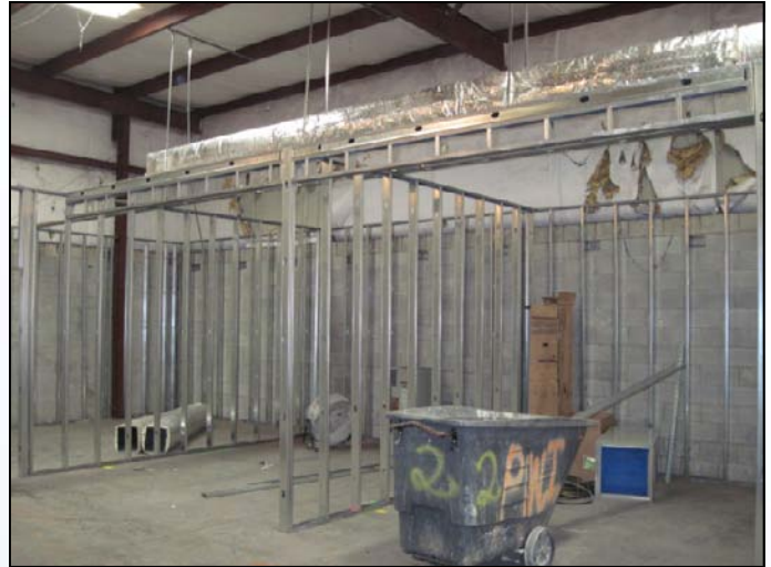
Frames for Walls Go Up December 14, 2009
