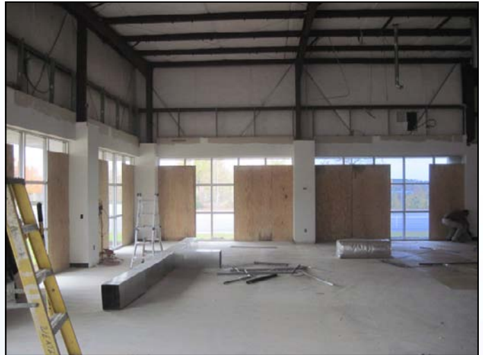
Renovations Begin on the Inside December 4, 2009
