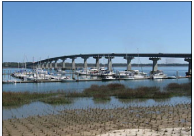
A parallel bridge will run along side the McTeer bridge when the project is complete.
