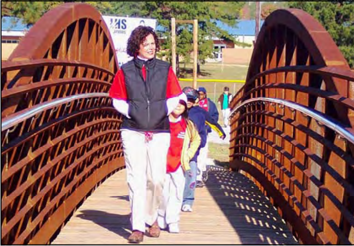
The Roddey Drive Pedestrian Bridge provides a safe crossing for students.
